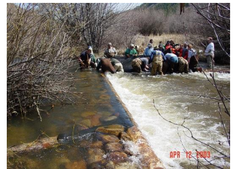
Building Plunge Pool on the North Fork of the Salmon River
