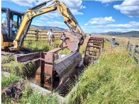
Diamond Creek Canal Fish Screen Install
