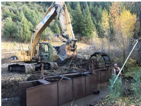
Travis Weeks Diversion Canal Fish Screen Install on Rainey Creek
